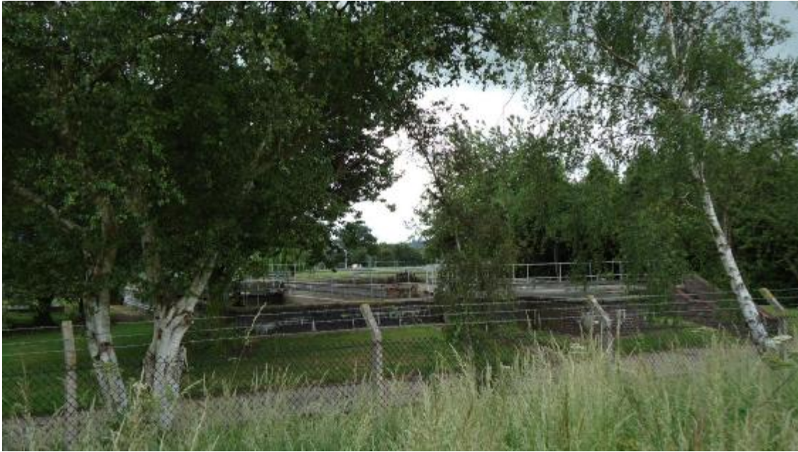
View east from The Dove Way to the sewage treatment works
