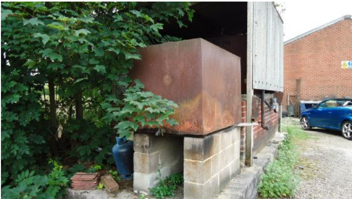
ASTs adjacent to the vehicle repair works
