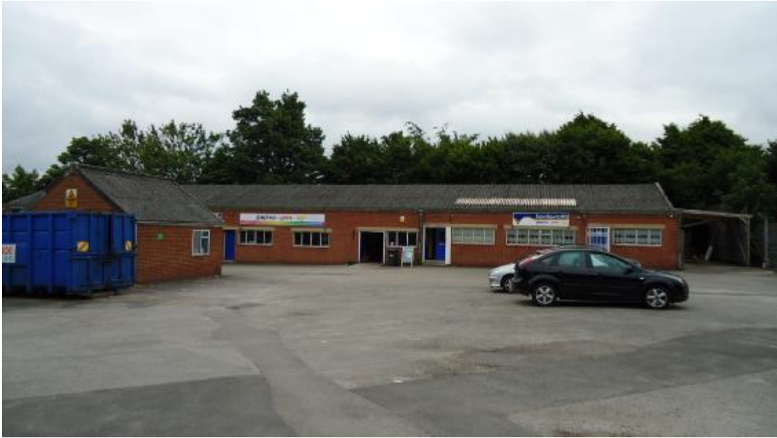
Industrial Buildings in the south of Area B
